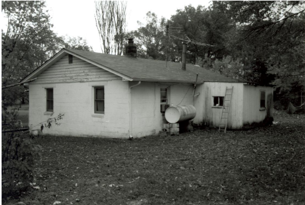
Figure 31 43035 Braddock Road, SW and NW Elevations in 2002
