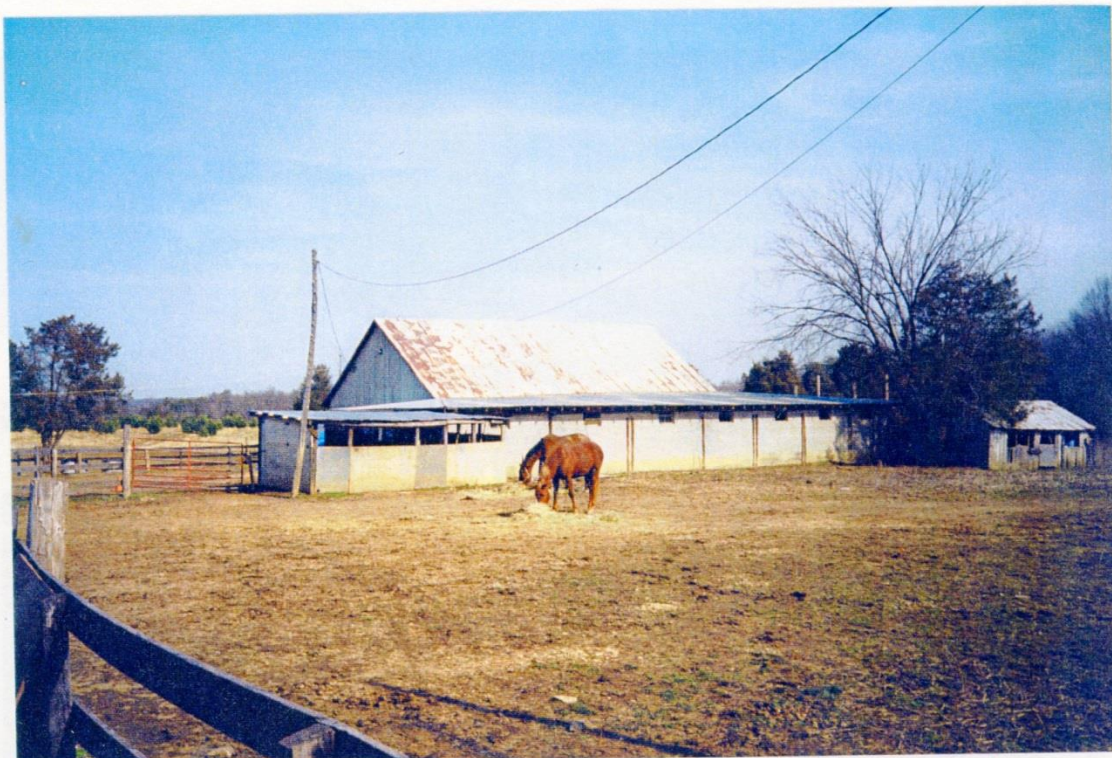
Photograph 20. View of stable building and the two storage sheds located at the southeast and southwest corners of the stable.
