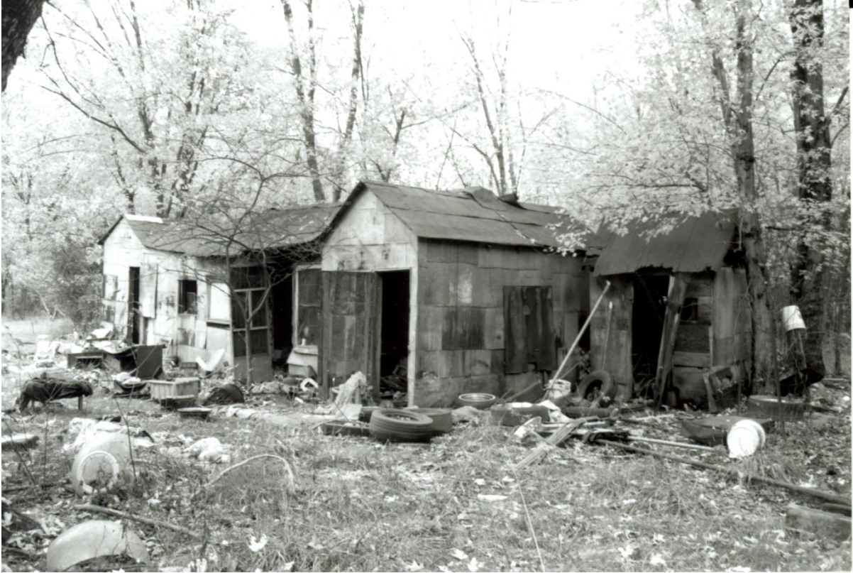
Figure 21 25974, Elk Lick, South Elevations, shed, West.
