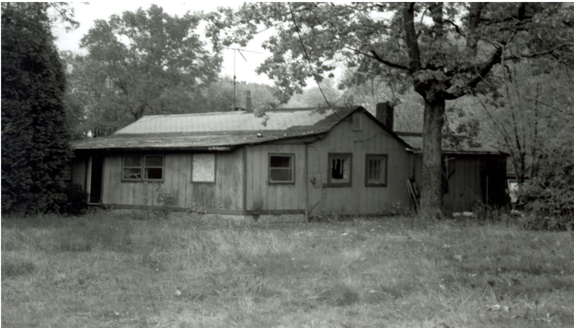
Figure 22 25974 Elk Lick, West and South Elevations
