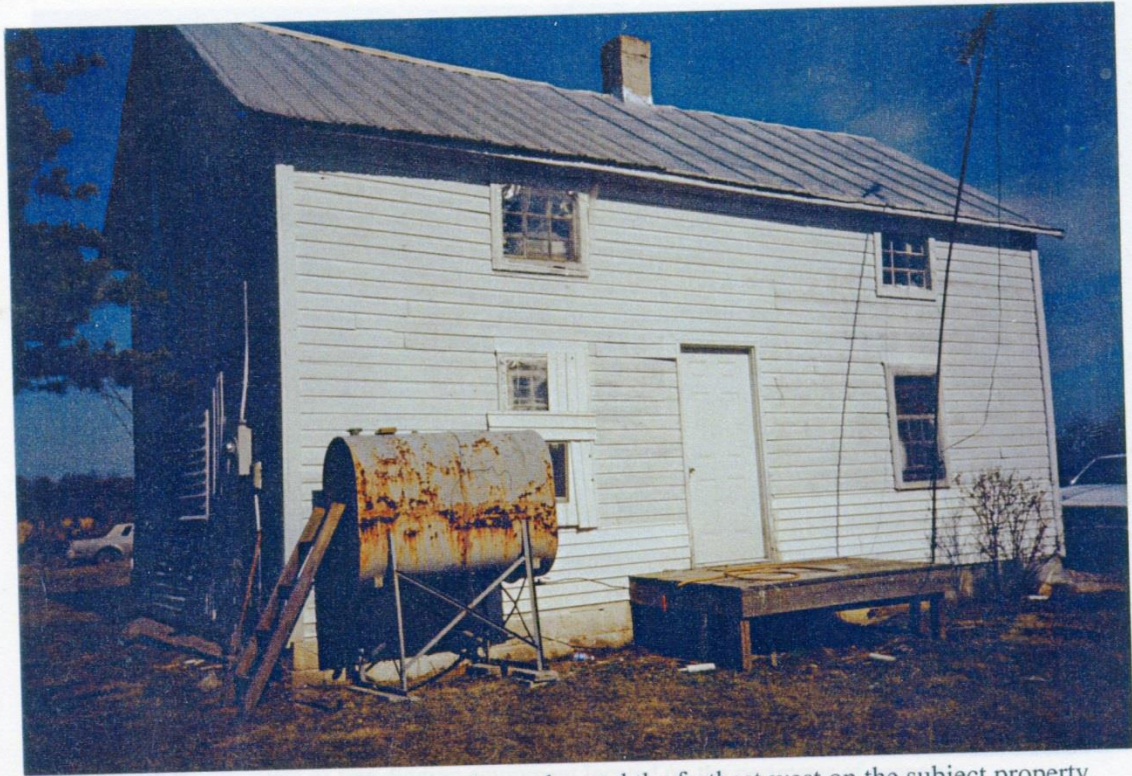
Photograph 7. View of the two-story house located the farthest west on the subject property.
