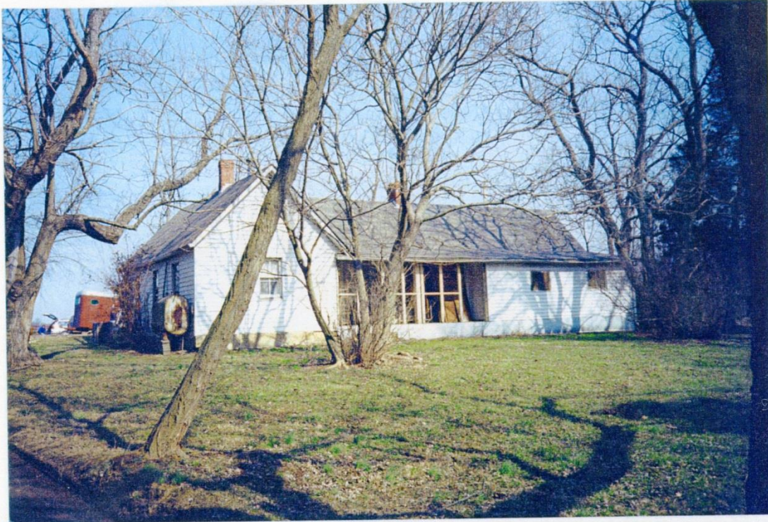
Photograph 19. View of the one-story residence that is part of the equestrian facility.
