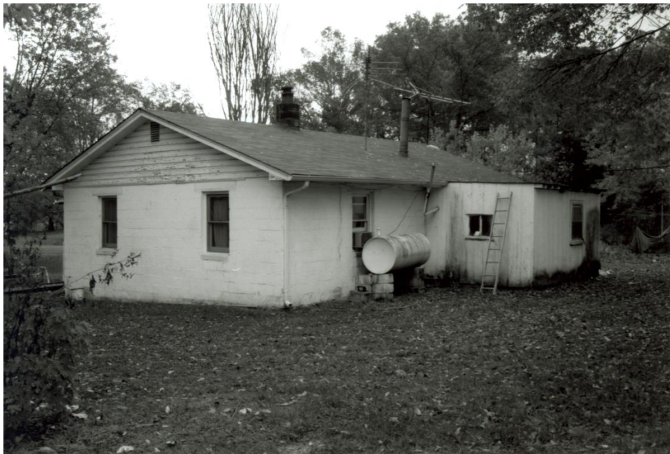
Figure 34 43035 Braddock Road, SW and NW Elevations in 2002
