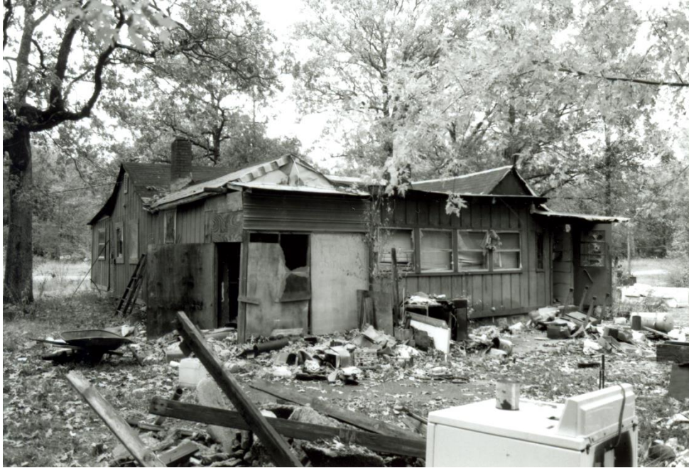
Figure 25 25974 Elk Lick, East & South Elevations, 11/6/2002
