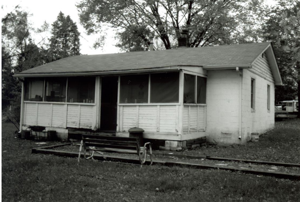
Figure 33 43035 Braddock, NE and NW Elevations in 2002
