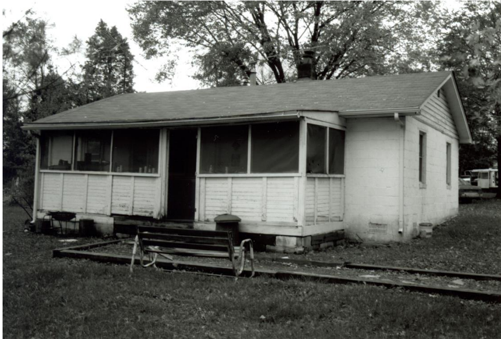
Figure 30 43035 Braddock, NE and NW Elevations in 2002
