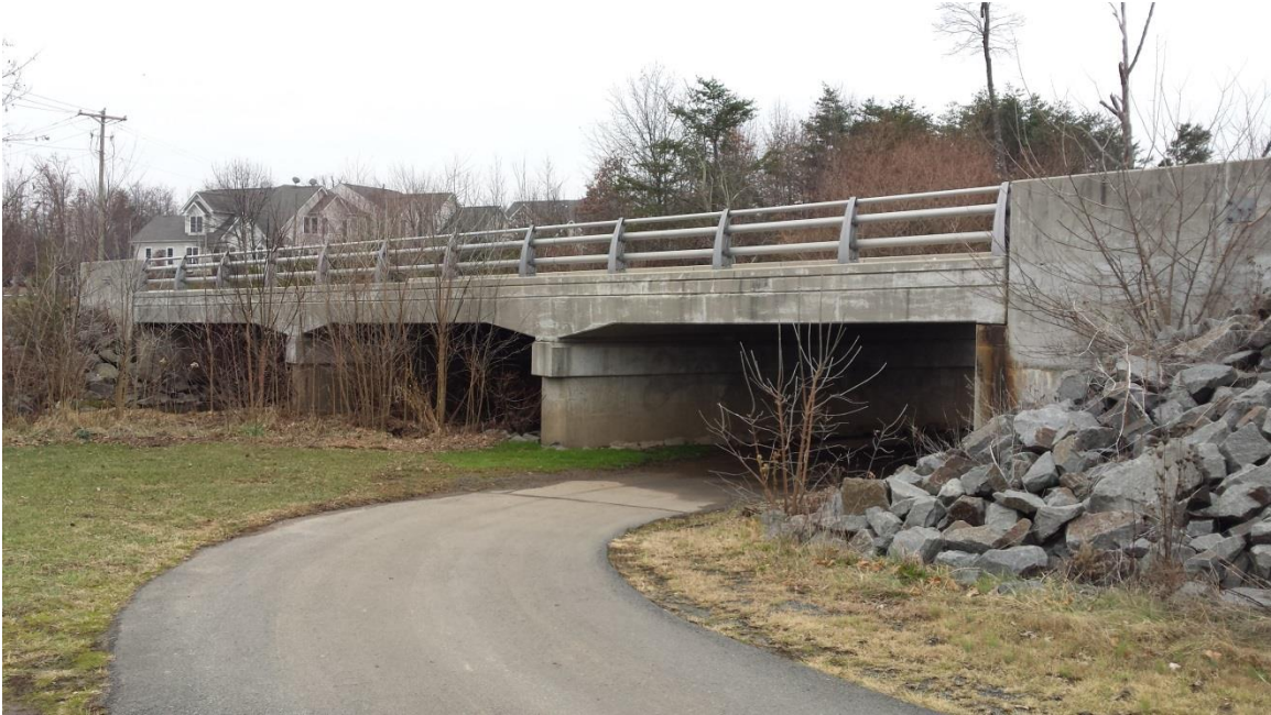
Figure 3 Elk Lick Road Bridge 12/1/2013
